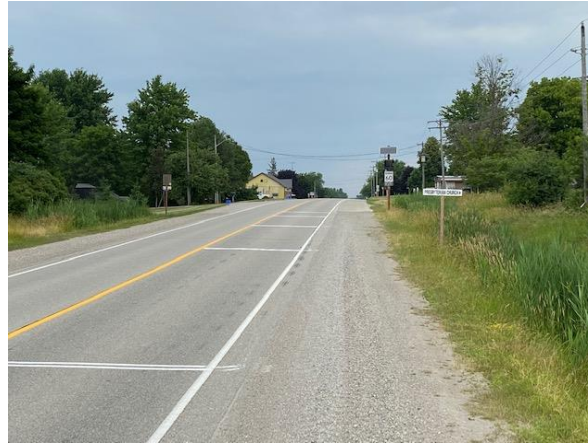
Transverse Bars (Uniondale)
