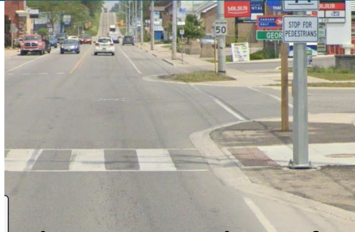
Curb Bump-out (Thamesford)
