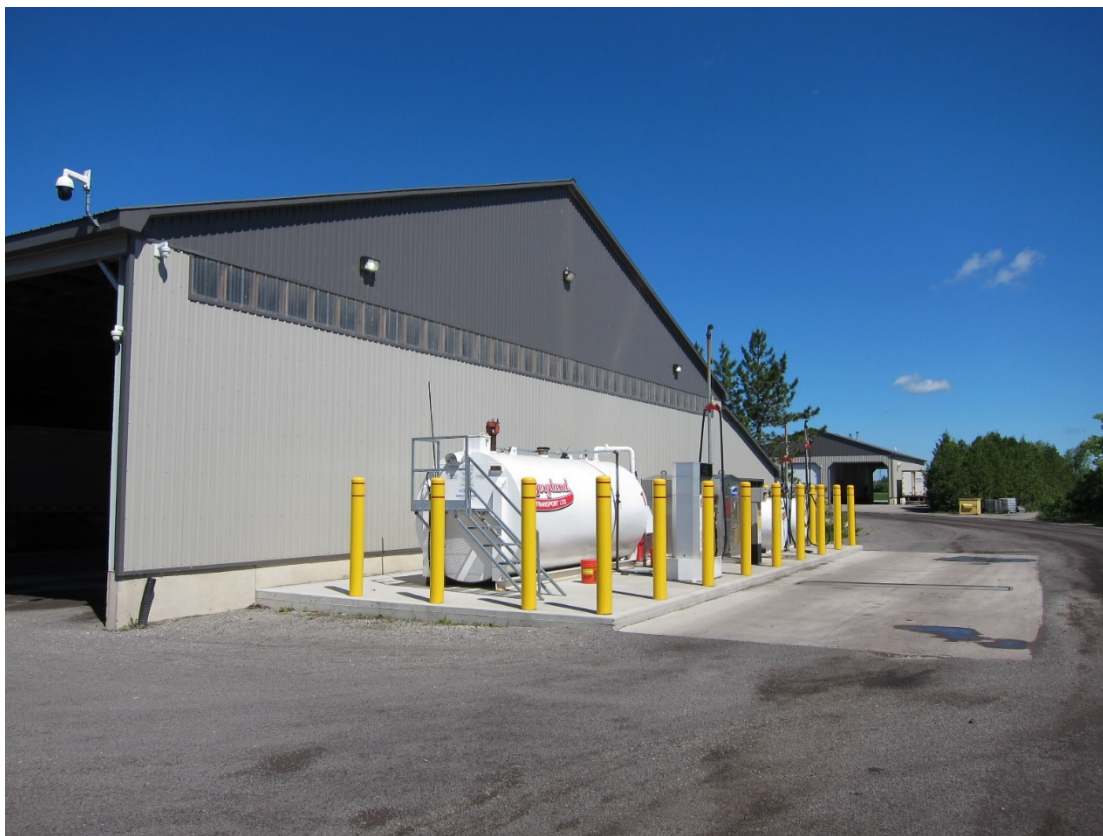
Photo No.4. View of both buildings (Building 1 in the background, Building 2 in the foreground).
