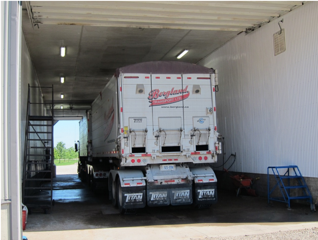
Photo No.2. View of south side of Building 1 – wash bay
