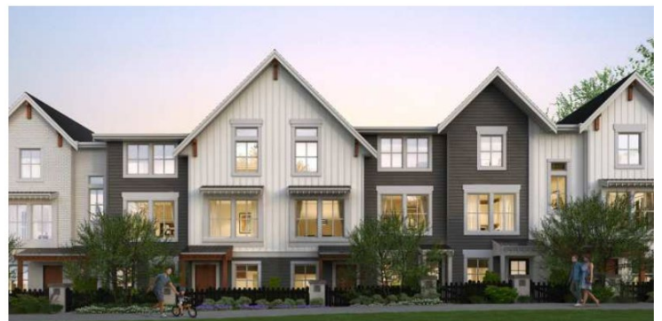
Street fronting townhouses (Image Credit: Gatehouse Developments)
