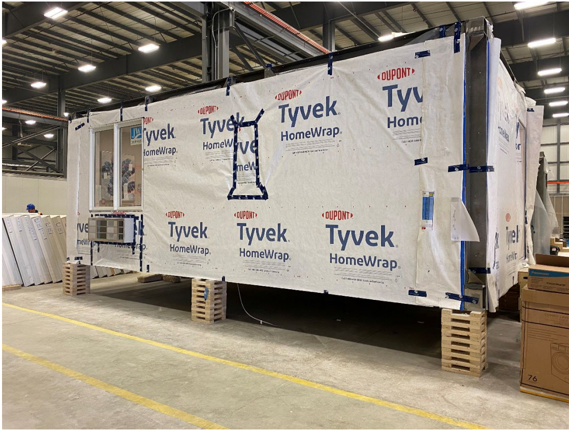
Exterior of modular unit under construction:
