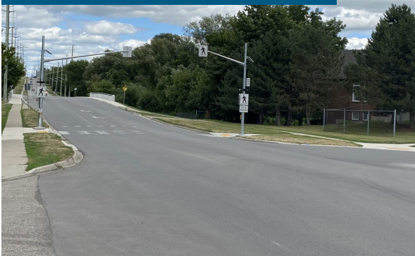
NEW PEDESTRIAN CROSSING – PARKINSON ROAD IN WOODSTOCK
