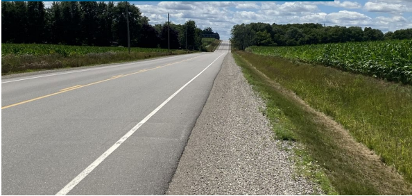
NEW SECTION OF OXFORD ROAD 16 – PHASE 1: RURAL ROAD WITH UPDATED CROSS SECTION, EAST OF KINTORE
